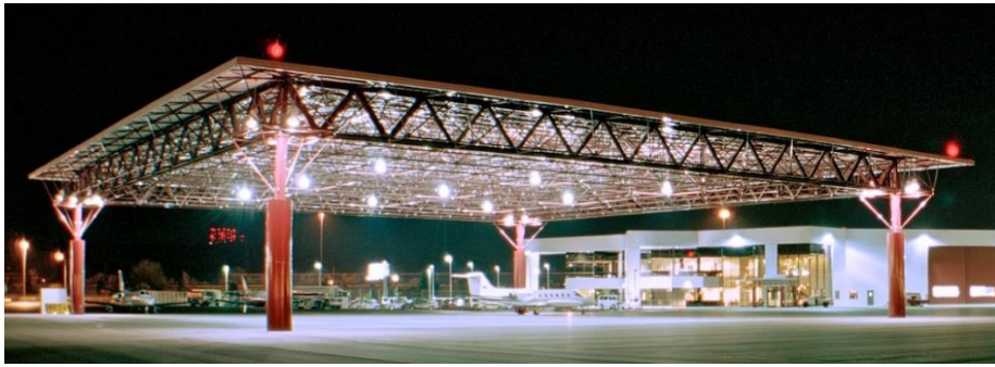
Fig. 13 An application of the grid structures [15].
