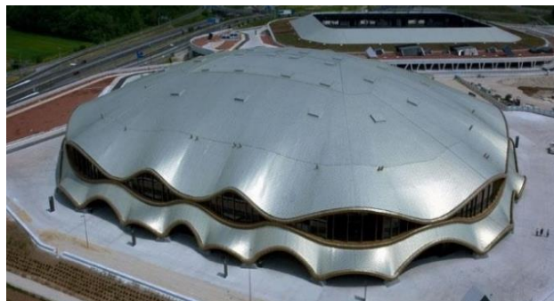
Figure 1. Multi-purpose sports hall (Slovenia)
