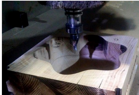
Figure 11. Block in wood at CNC machine for generating A scallop dome formwork
