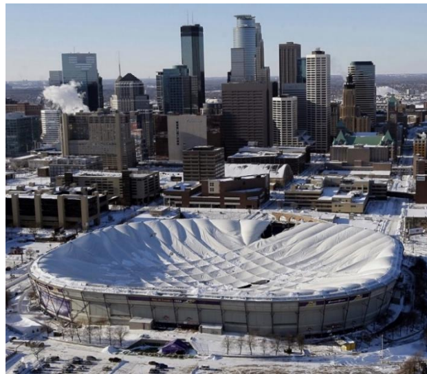
Figure 4. Collapse of the American Metro Stadium resulting from storm and wind
